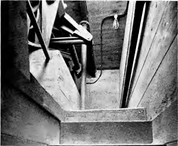
Fig. 155—Entrance Way into the Foundation Pit of a Jolt-Moulding Machine, showing Steps leading into the Pit from an Adjoining Basement Room.
